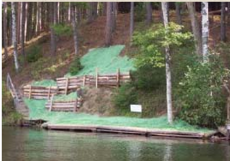
Below: The completed LUNKER with additional bank stabilization practices, including terracing, revegetation and the placement of a mulch blanket.
