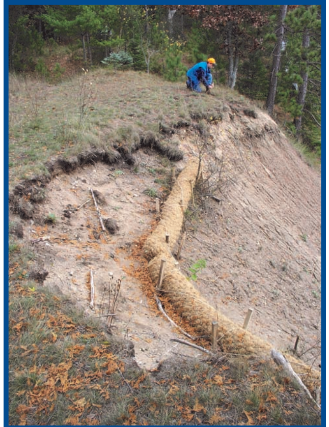
A coir log helps to stabilize Claybanks, a severe erosion site.
