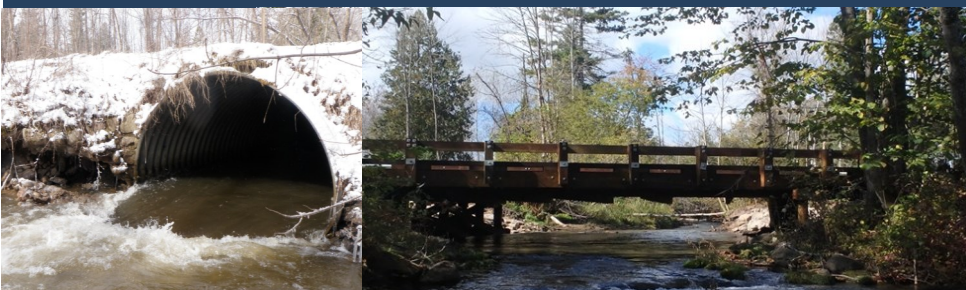
New timber bridges at Houghton Creek (before and after shown) & the E. Branch Au Sable have opened up river habitat & improved community infrastructure.
