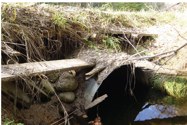
Crump Road culvert on Mullett Creek - Before
