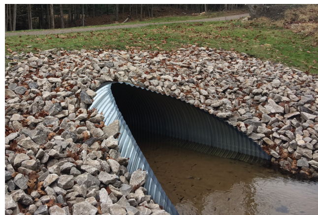
Crump Road culvert on Mullett Creek- After
