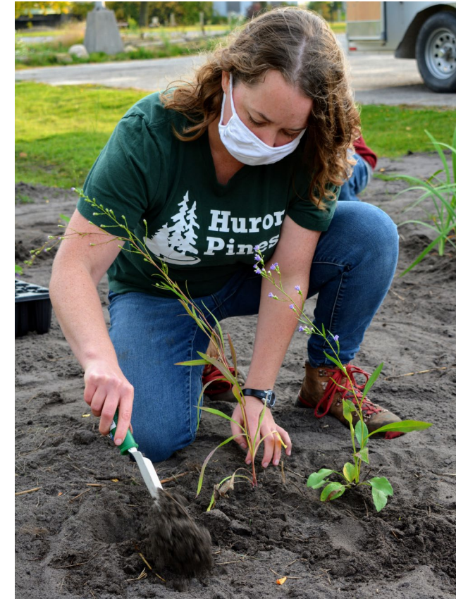
Water Program Director Samantha Nellis situates native plants in a bioswale designed to capture and filter stormwater at Au Gres Riverside Park.
