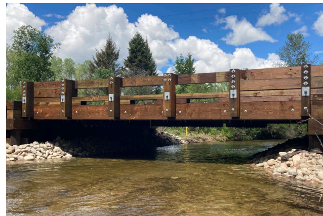
The new timber bridge spanning Gilchrist Creek.
