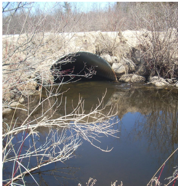
The former culvert at the Shingle Mill Crossing.
