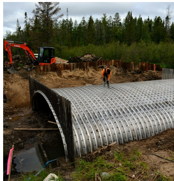
The new 27-foot arch structure during the installation phase.
