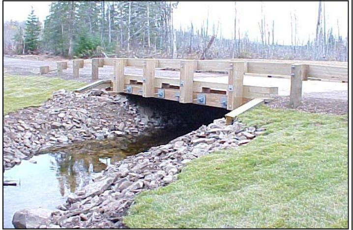
Above: This timber bridge in Cheboygan County was completed Winter 2003. This project improved fish passage and reduced the amount of sediment entering the stream.
